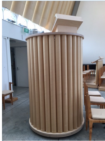
Pulpit, constructed of smaller cardboard tubes
