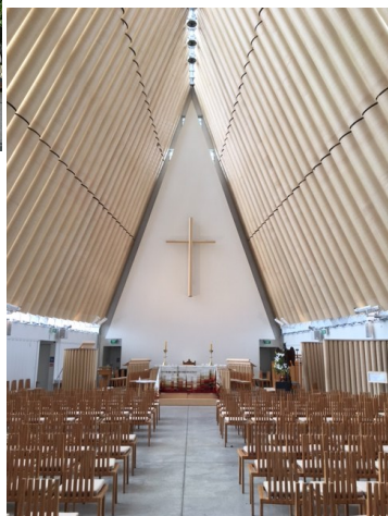
The cathedral’s A-frame interior, made of massive cardboard tubes
